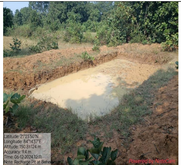
Recharge Pit at Beheramal,Sambalpur
