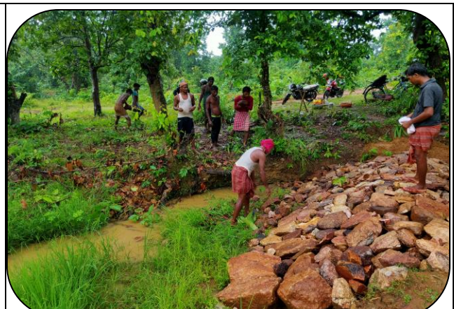
Loose Boulder Structure At Tampargarh, Sambalpur
