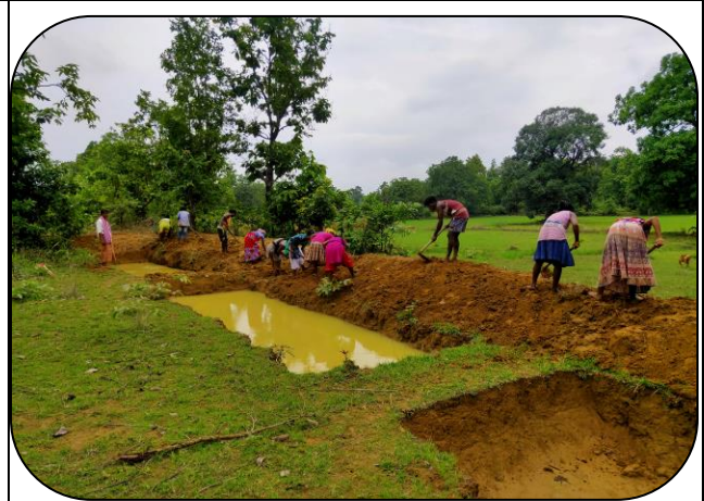
Water Absorption Trench (WAT) At Tampargarh, Sambalpur
