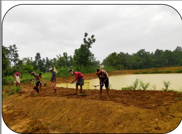
Farm Pond At- Beheramal, Sambalpur
