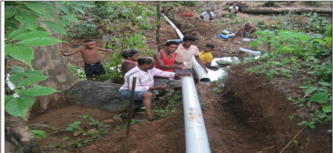
Laying of Pipe Of DBI Project At-Kristianpada,Rairakhol,Sambalpur
