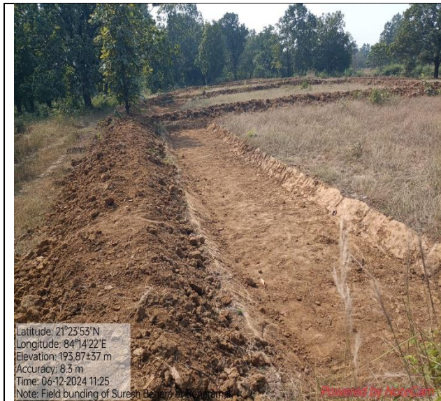
Field Bunding at Beheramal,GP- Tampargarh,Sambalpur
